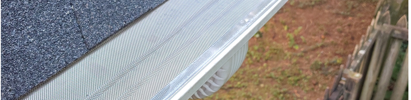
Stainless-steel mesh and aluminum edges on a real Clean Pro installation.
