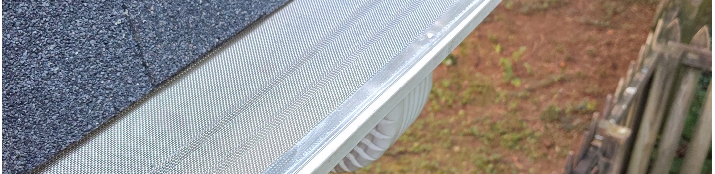
A real Clean Pro Guard installation. Stainless-steel mesh with aluminum edge bands.
